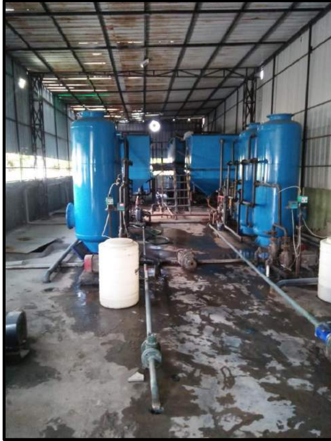
Sewage Treatment Plant
